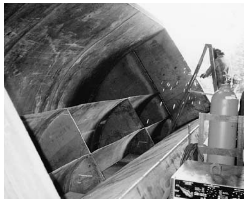
Welding of 45° flue elbow.
